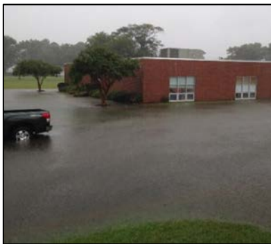
Figure 3: Flooding at Westhaven Elementary School, September 2014
